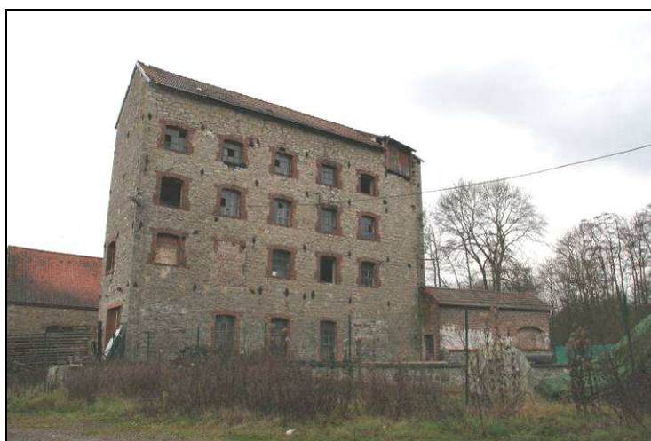
Figure 31: Tannerie de Dourbes (Photo: AWP+E)
